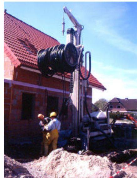
Photo 1. Installation of borehole heat exchanger at a small house in Bielefeld, Germany, using a small, powerful Rotomax drilling rig.
